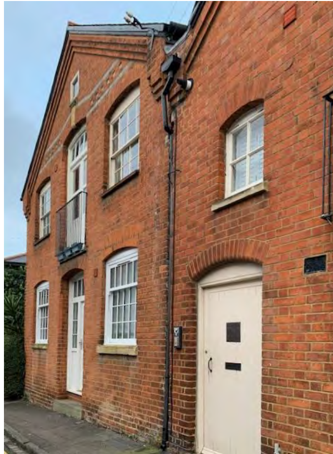
Figure 32: Conquest Court, a residential conversion of a former light industrial premises (image Evelyn Williams)
